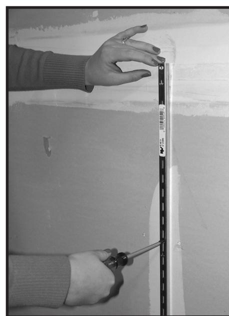
Using a drill with a 1/8 in. bit, drill a hole 2 in. deep on the mark you made in step 2. Line the middle hole of the wall bracket up with the hole and insert a wall bracket screw. Leave the screw loose for now.
