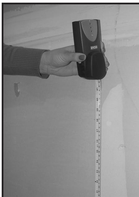
Using a tape measure, mark a spot on the wall 36 in. from the floor. This will be the location of the middle mounting hole and screw for the wall bracket.
