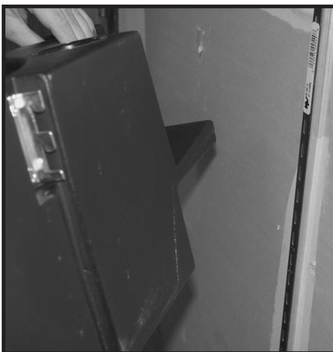
Line up the standard guide and mounting bracket on the Vac Station. Mount the vac station at the proper height. You may need to loosen the three mounting screws a little if the bracket doesn't slide into a secure fit.
