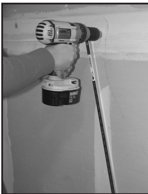
Rotate the wall bracket to the side and with the same 1/8 in. bit, drill two more holes 2 in. deep, one on each of the marks you made in Step 4.
