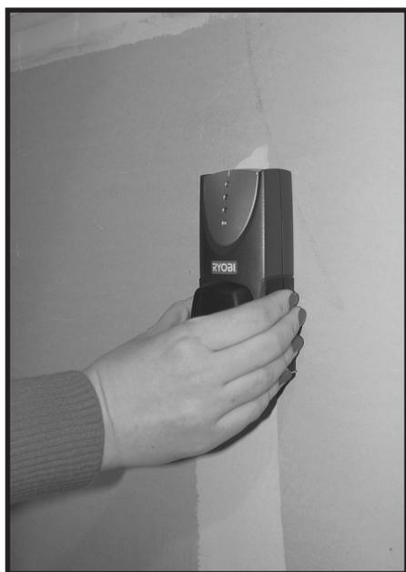
Using a stud finder in the area you wish to mount the ProTeam Vac Station, locate and mark a wall stud. Be sure to mount the Vac Station into a stud, not just the wall board or sheet rock.
